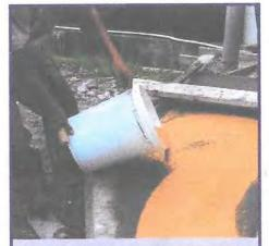
Mix the KG Colour Cement slurry with approximately 38% water using an electric stirrer. Pour the slurry to the substrate.
