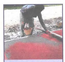
Powder the dry KG Colour Cement powder on to the fresh concrete or floor screed. Sprinkle about two thirds of the needed powder for the surface in the first layer.
