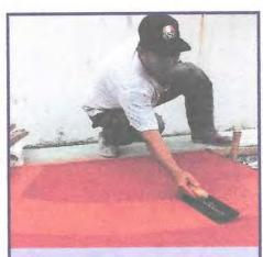
Let the colour cement absorb the water from the substrate for a short while, then float the surface thoroughly. When completed 1'st coat sprinkle the remaining cement for the 2'nd coat and float it. If needed add a bit of water to the surface.
