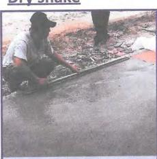
After initial setting when concrete / screed is still soft the colour cement can be added.
