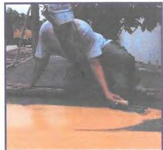
Spread the slurry with steel trowel to an even surface. Usually minimum two coats are needed.
