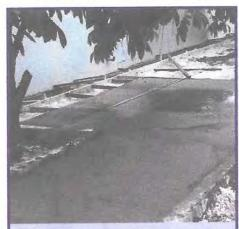
Let the fresh concrete or floor screed harden up to touch dry condition. Usually 2-4 hours dependent on climatic conditions.
